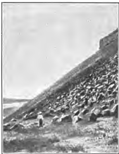
FIG. 25. — The destruction caused by freezing water.
